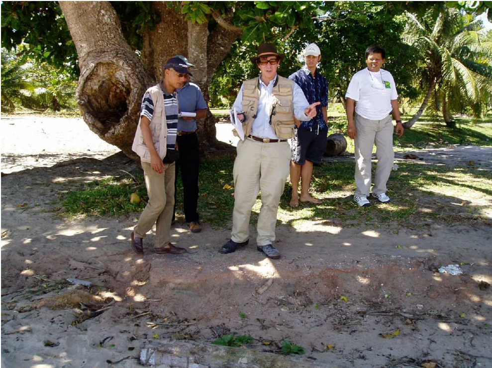
Figure 4. Scouring of a road along Ampandrozonana Beach in Sambava (Site 6). Top Left: General view of the beach, with the eroded road segment to the left, 71 m away from the water line. Top Right and Bottom: Close-up of the scouring. Note the advance of the beach, identified by sand deposits, over the previous location of the road.
